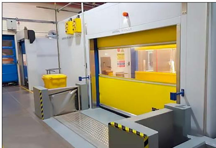
The Anhamm barrier is FM Approved for flammable liquid retention.
