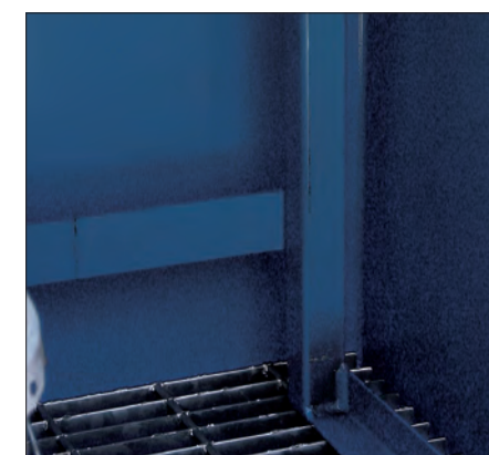
Bottom supports rest directly on grating.
