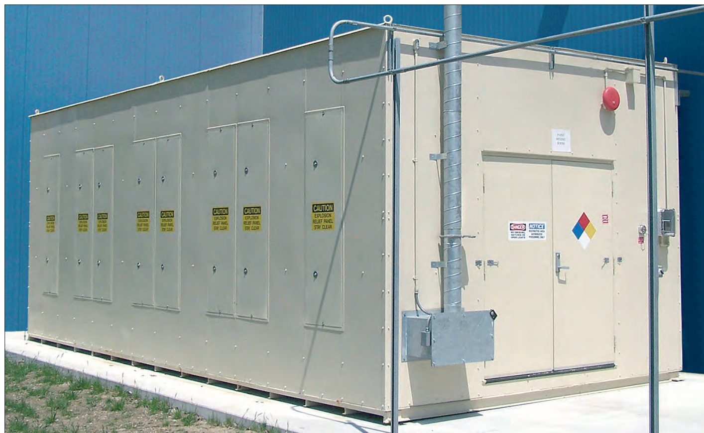
Heated and cooled storage Occupancy Building with fire suppression system, fire rated construction, and explosion-relief panels designed to house automotive paint pumping equipment.
