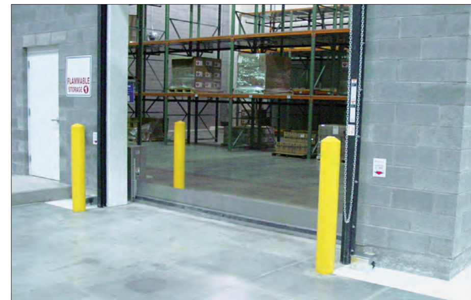
Automatic Doorway Spill Barriers are often utilized as containment equipment for Flammables Storage Rooms
