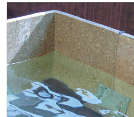
Segments seal together to form a virtually leak-proof barrier
