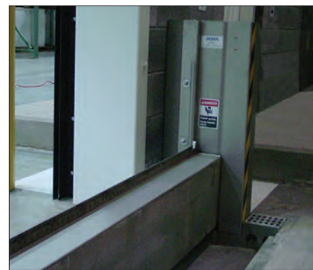
Doorway Flood Barrier in closed position.
