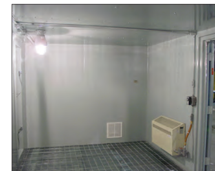
Interior of Occupancy Building shows electric heating unit, explosion proof light, and XP controls.
