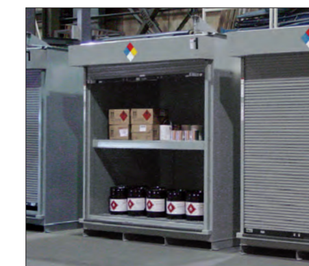
Fire rated Locker modified to have two levels. Used to store small volume containers of flammables.
