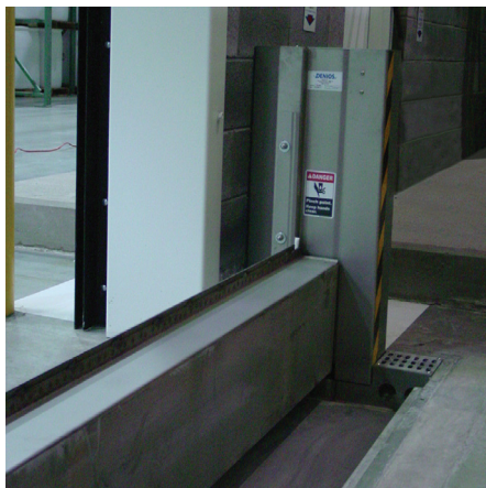
Doorway Flood Barrier in closed position.
